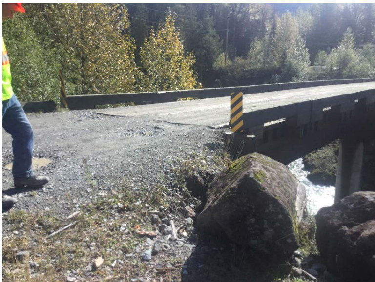
Right Bank Abutment when facing downstream
