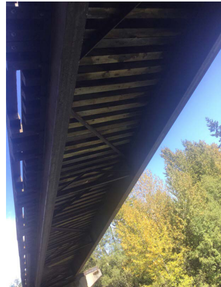
Main span superstructure
