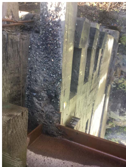
Main span, left abutment sill - downstream side
