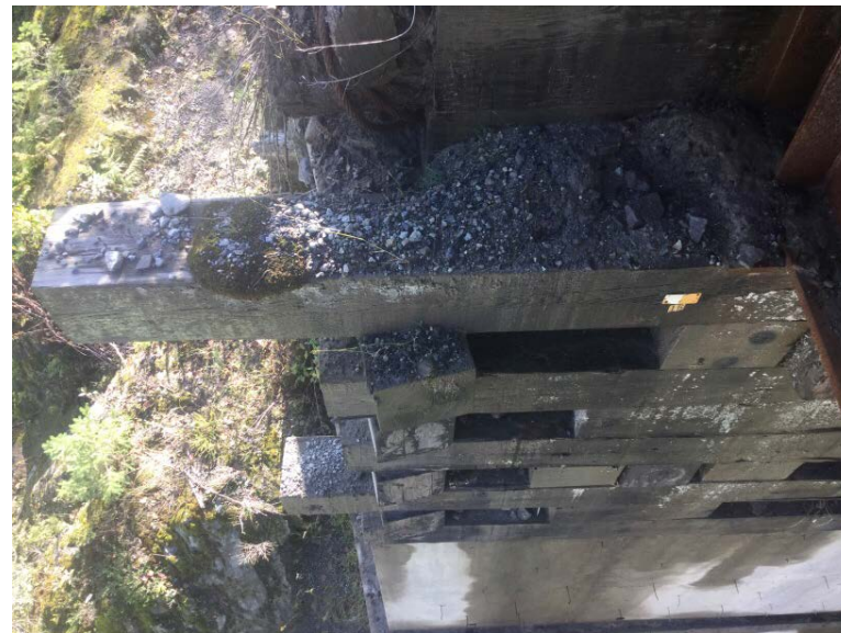
Main span, left abutment sill
