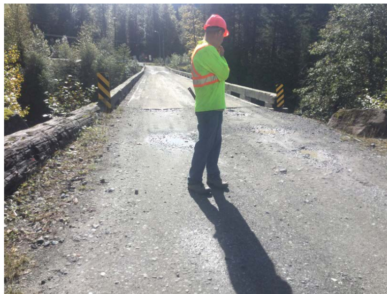
Right Bank Abutment when facing downstream
