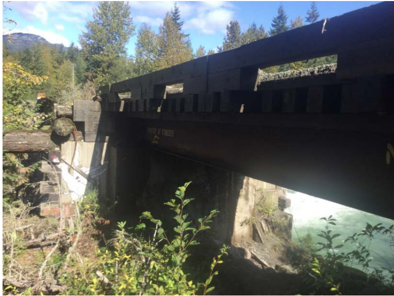
Left Bank Abutment when facing downstream
