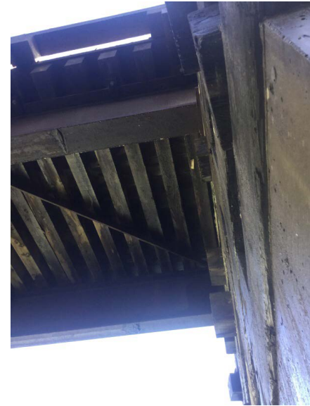
Left pier, stream side
